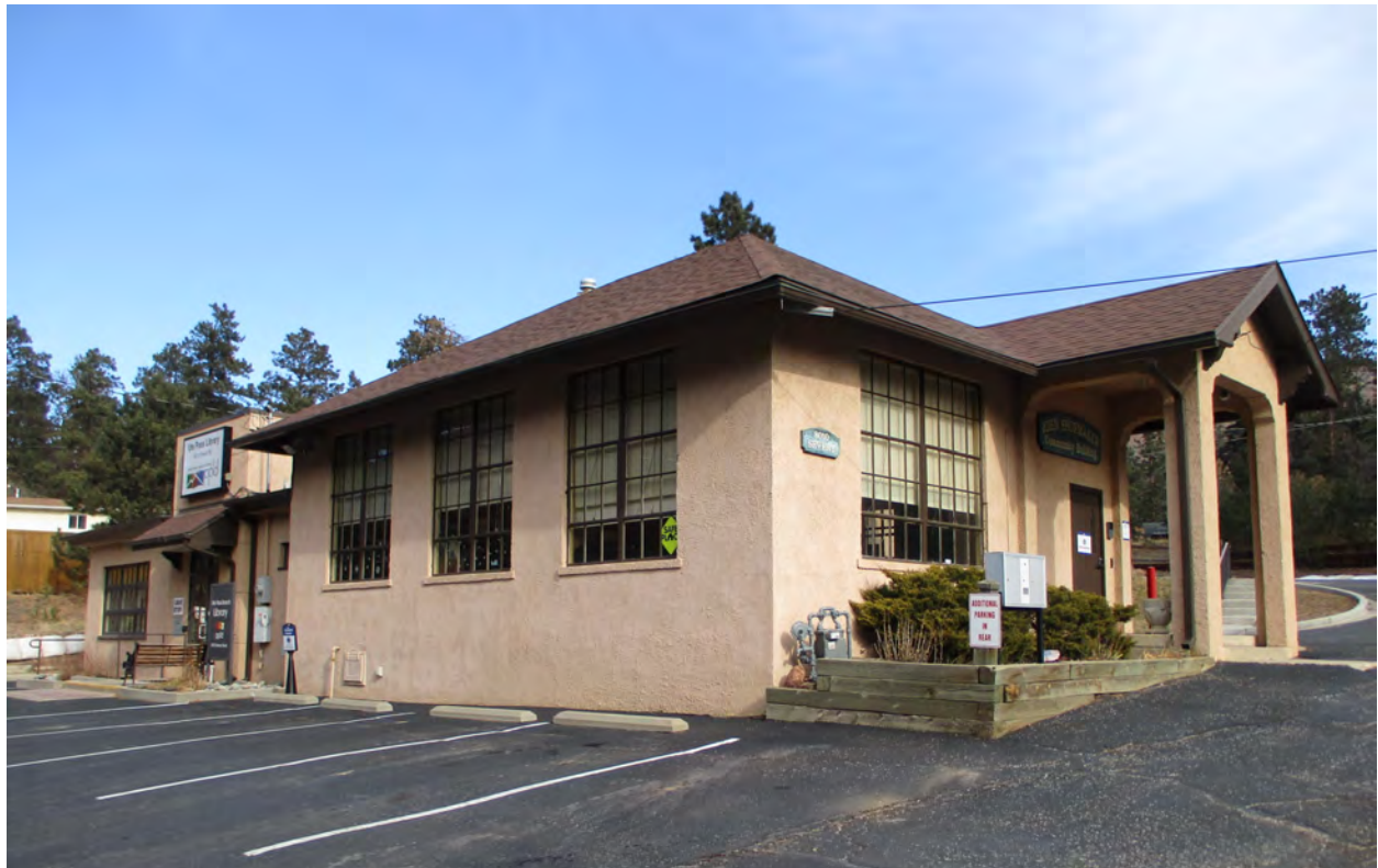
SUBJECT LOOKING NORTHWEST
